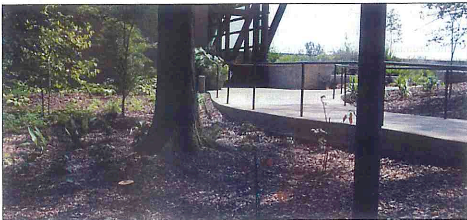
This root bridge protects the trees along a sidewalk entrance. Arborguard also used a compactible fill material over root systems for walkway areas to protect the soil profile, so it retains the ability to exchange gas or water.
