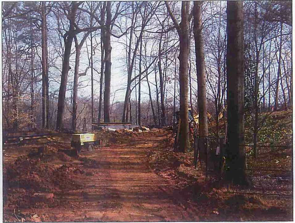
Protective fencing was going up around the trees along a roadway during early construction, above, and was still in place nearing the end of the job, below.
