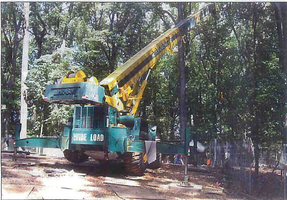
Altumnats ground protection pads were used to protect the root zones as much as possible, as shown above.
